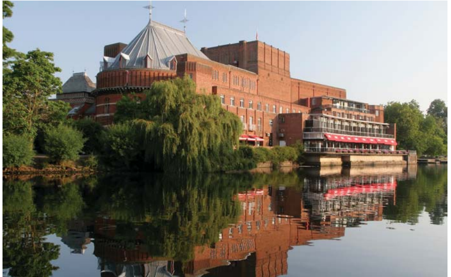
Mace Group is construction manager on the Royal Shakespeare Company's theatre transformation project which involves partial demolition and rebuild of the Grade II* listed theatre to provide a thrust stage auditorium
